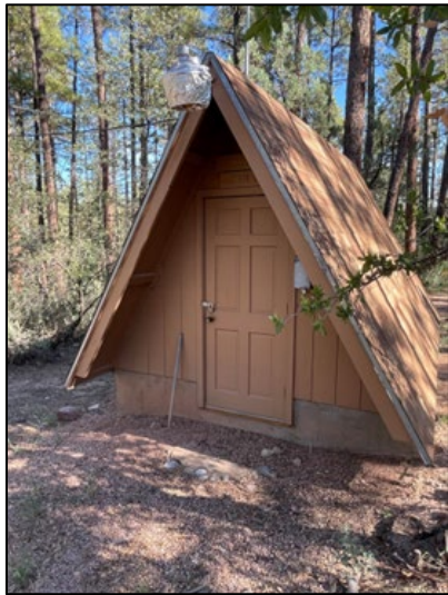
VG2 Facility (Booster pump and bladder tanks)
